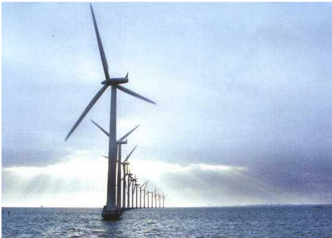
Offshore park Middelgrunden, Denmark, 20 2MW Turbines
