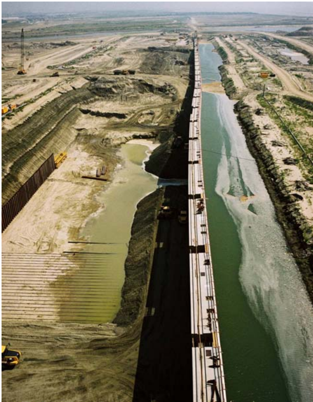
Retention wall and flooded ditch
