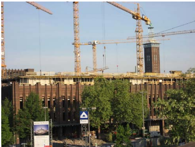
Total internal renovation of an existing office building
