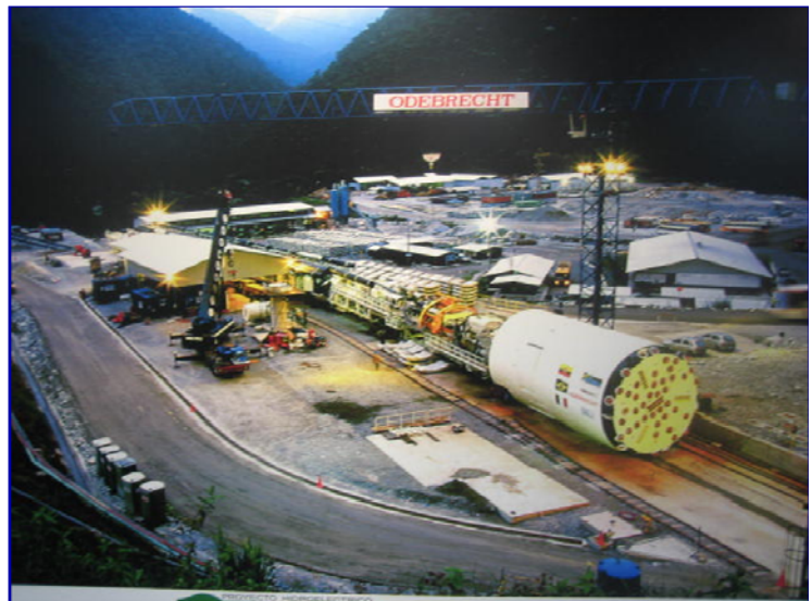
Picture depicting the tunnel boring machine and back-up train during assembly
