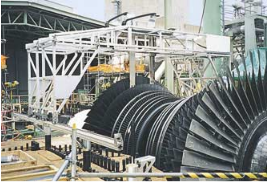
Figure 22 Seven-axis robot during disk examination of an LP turbine shaft in the assembled condition
