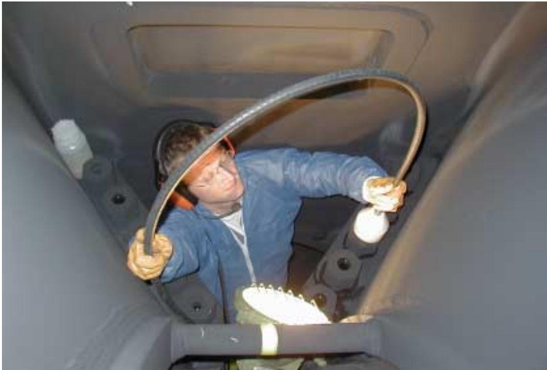
Figure 28 System for inspection of casing joint bolts
