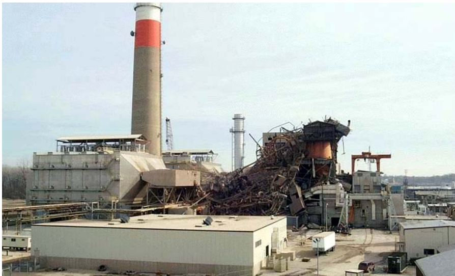
Figure 1 – Boiler Explosion
