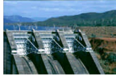
Spillways associated with embankment dams are independent or “stand alone” concrete channel structures located on the slopes of the river valley.
