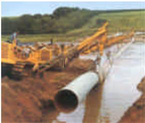
Wide river crossings involve several cranes, possibly pontoon mounted units to carry the pipeline over the whole width of the river. The pipeline is then laid in the trench simultaneously by all cranes in tandem. Since one unit alone cannot support the weight of the pre-welded pipe section this operation is difficult to ensure none of the units become overloaded and topple or capsize into the river.
