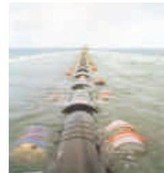
This 'standard' method can be used for depths of up to approximately 100 m whereby the progress rate under normal conditions is about 1.5 – 2 km per day. For depths over 100 m., other methods have been developed which fall outside the scope of this paper.
