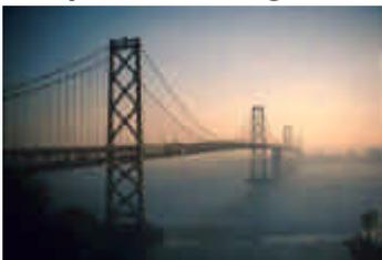
Suspension bridges are often very “slim” structures, principally comprising of pylons, main bearing cables, hangers and bridge decks. The design lends itself well for both relatively short spans to 1.500 m and longer.
