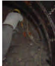
3. Drill and Blast The technique is exclusively used in rock tunnels where the ground conditions are sufficient for the already completed sections to resist against the blasting vibrations. The stand-up time of the unsupported span must also enable installation of any support systems that may be required - or otherwise in accordance with the NATM philosophy (described below).
