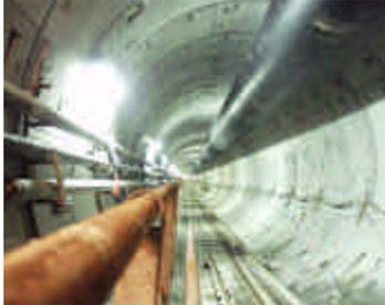
2. Jacked concrete pipes Used exclusively with TBM or shield drives. Instead of being installed at the TBM similar to segmental linings, they are installed at the start shaft and jacked into the tunnel to "follow" the TBM. Thus during the jacking process the whole tunnel moves forward as the TBM progresses.
