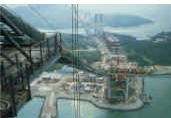
The foundations for the towers and the main –cable anchorages are completed first, followed by the towers/pylons from which the cables are hung (*as left*). The bridge deck is then suspended from the cables (*right*).
