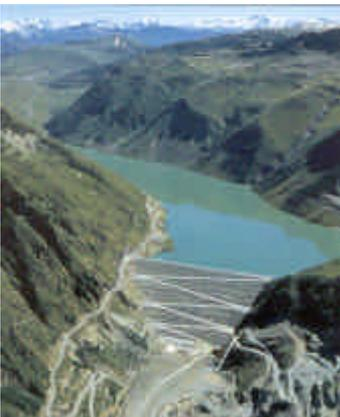
Embankment dams mainly include rockfill and earthfill dams. Earthfill dams can be either zoned - involving selected areas of rock, gravel, earth and impervious zones - or homogeneous. They do not need to be built on rock, and are not vulnerable to “soft” foundations such as decomposed rock or alluvial deposits.
