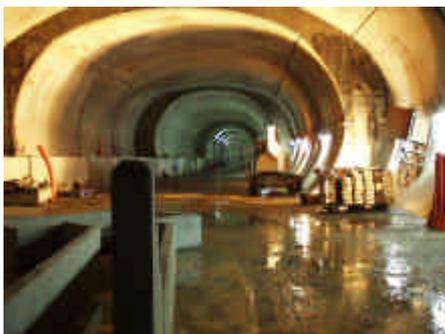
separate drives each reaching a state of equilibrium before the next is begun. This allows the ground loads to be progressively redistributed, into and around the lining, with
