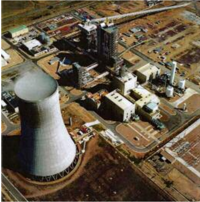
IGCC at Puertollano
