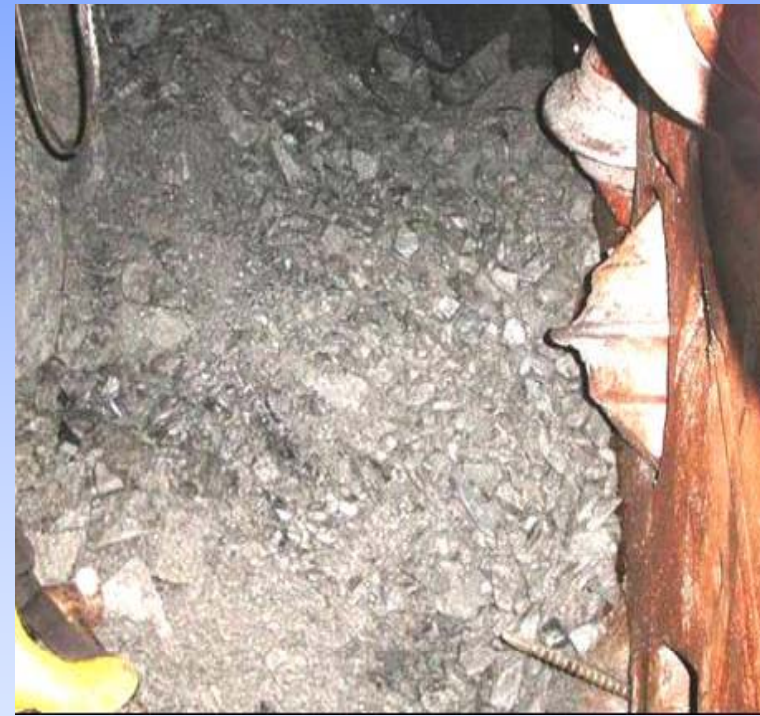
Fragmented rock from fault zone on RHS
