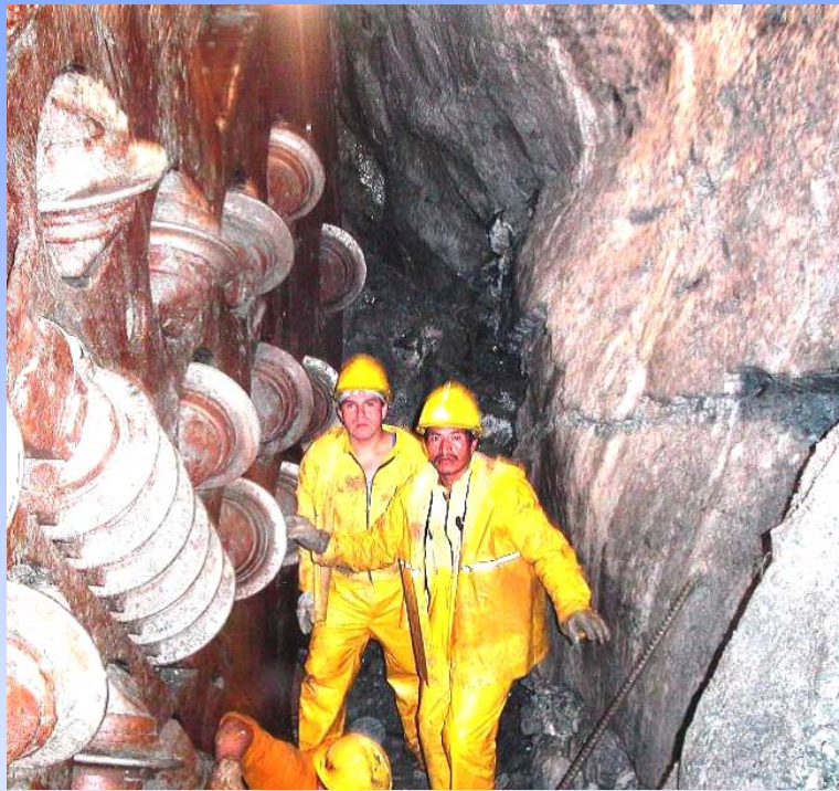
Cutter-head of TBM after removal of rock fragments, LHS stable
