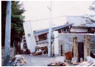
Collapsed 2-story wooden house
