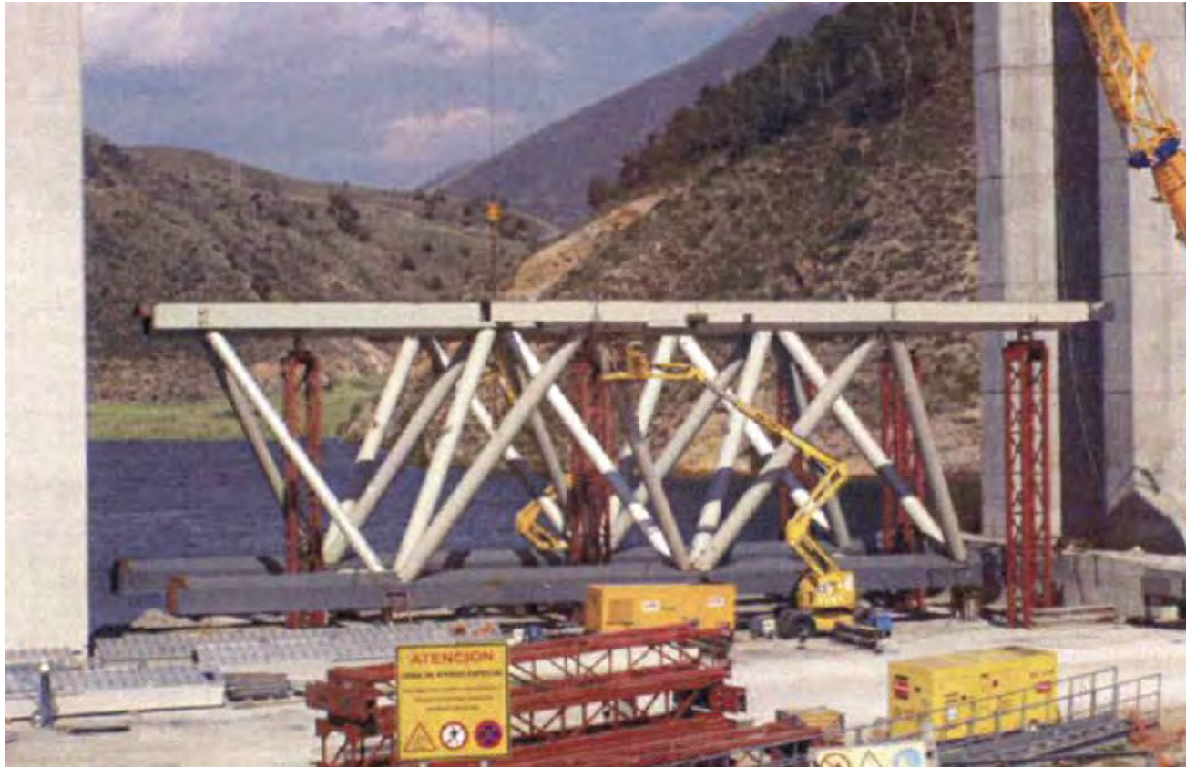
Preparation at ground level
