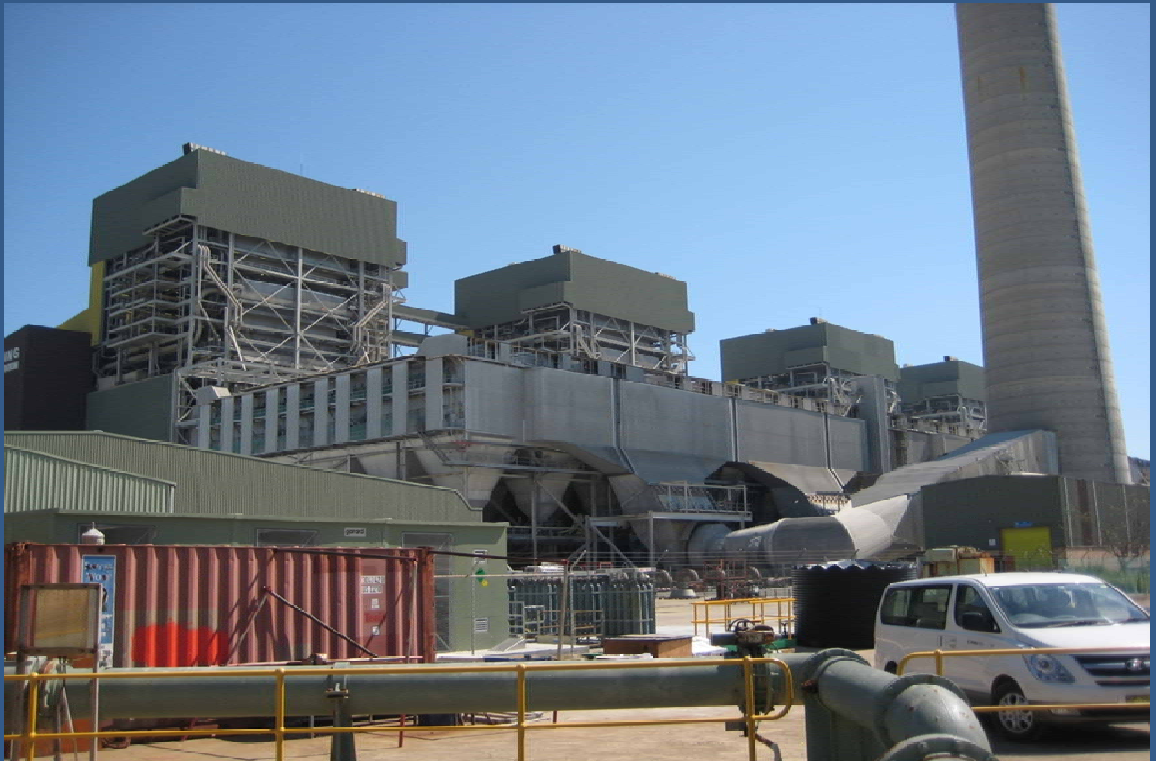
Coal Fired Power Plant, Australia
