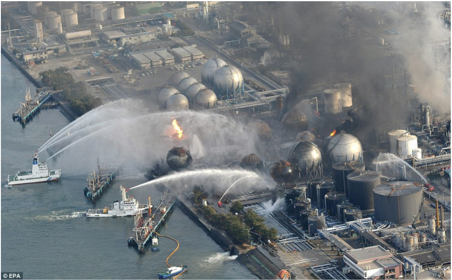
Ships try to extinguish a blaze at oil refinery tanks in Ichihara, Chiba Prefecture, which has been burning since Friday's earthquake and tsunami
