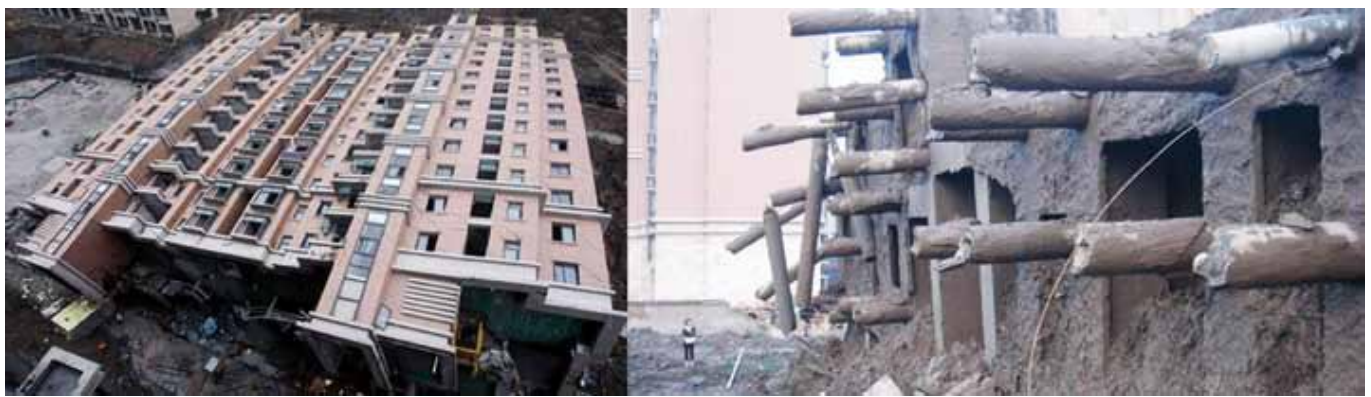
Figure 9. Toppled apartment building, Shanghai, 2009.
