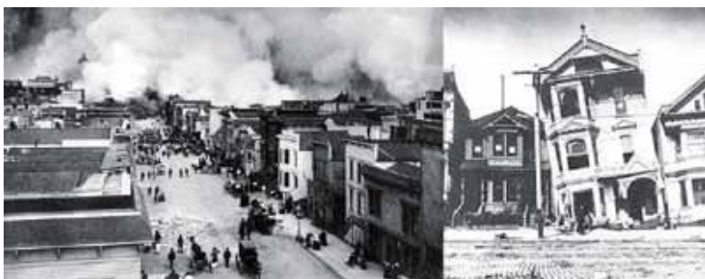
Figure 2. Typical damage in Bay Area, San Francisco (1906)
