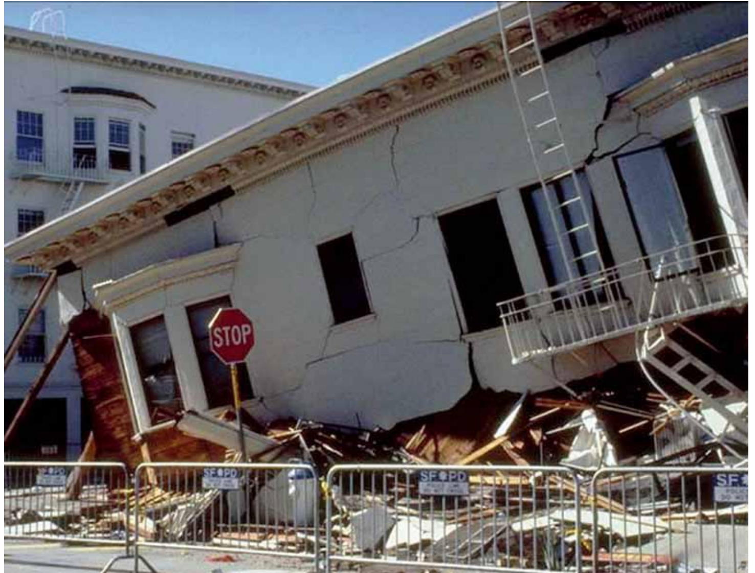
Figure 1. 1989 damage in the Marina District, San Francisco.
