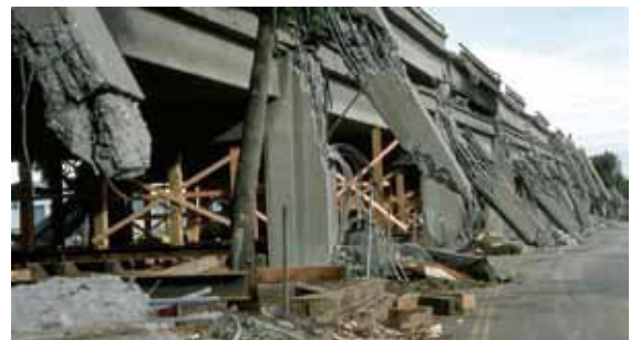
Figure 3. The Cypress Freeway after the 1989 earthquake
