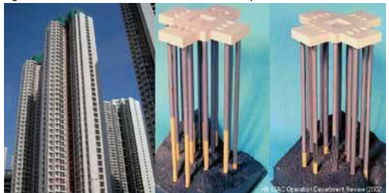
Figure 8. The tower blocks and models of their piled foundations.
