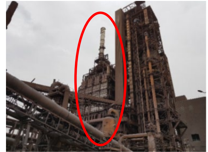
Process Gas Heater (left) DR Reactor (right) Courtesy of Emirates Steel (ES) Abu Dhabi UAE
