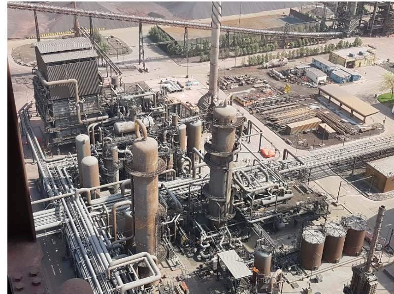
Courtesy of Emirates Steel (ES) Abu Dhabi UAE
