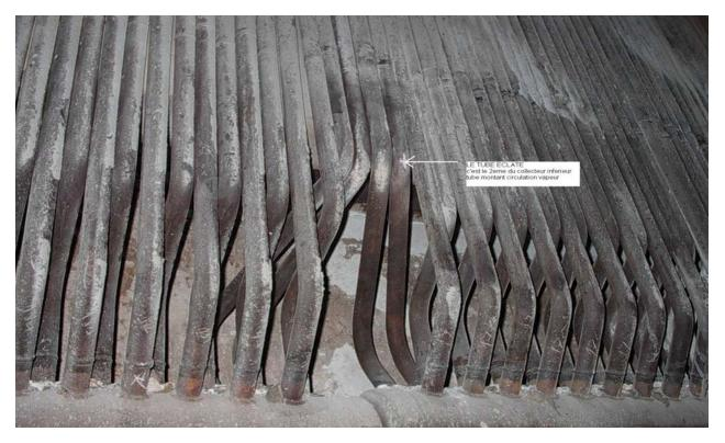
This pipe had been installed in order to collect condensate vapour, but no drain pipe has been observed.
