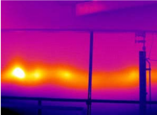
Figure 15 - Coal Silo Thermographic Image
