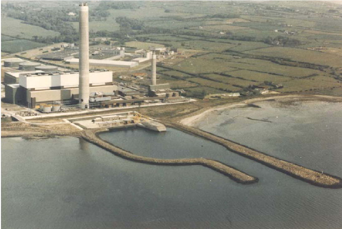
Photograph 6: Inshore Intake at Kilroot, Carrickfergus
