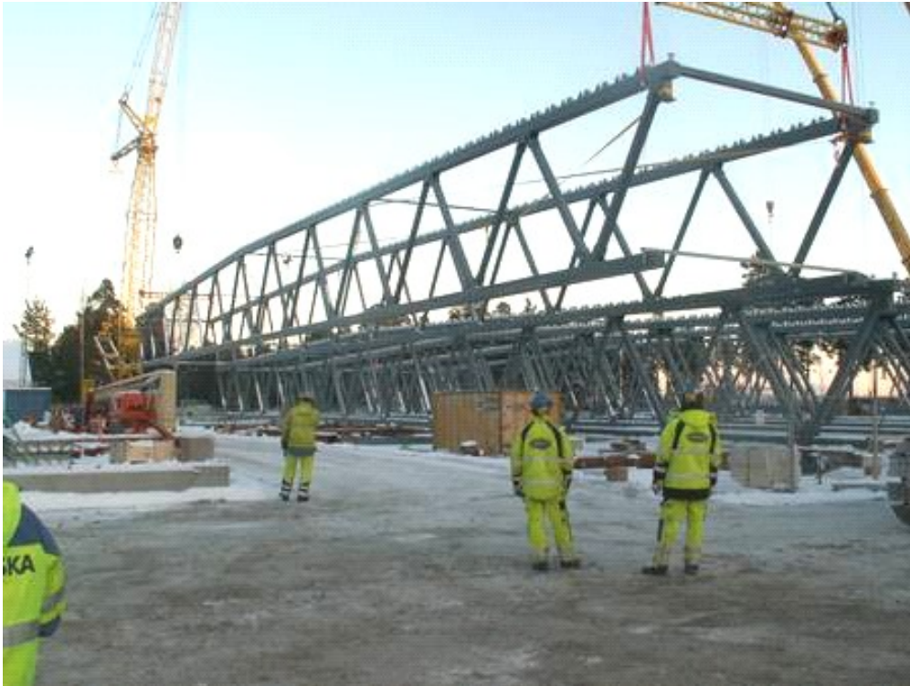
Picture 1 - Frame constructions
