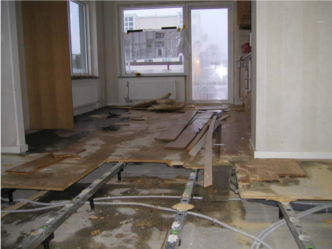
The similar view during stripping out of internal floors and other fittings
