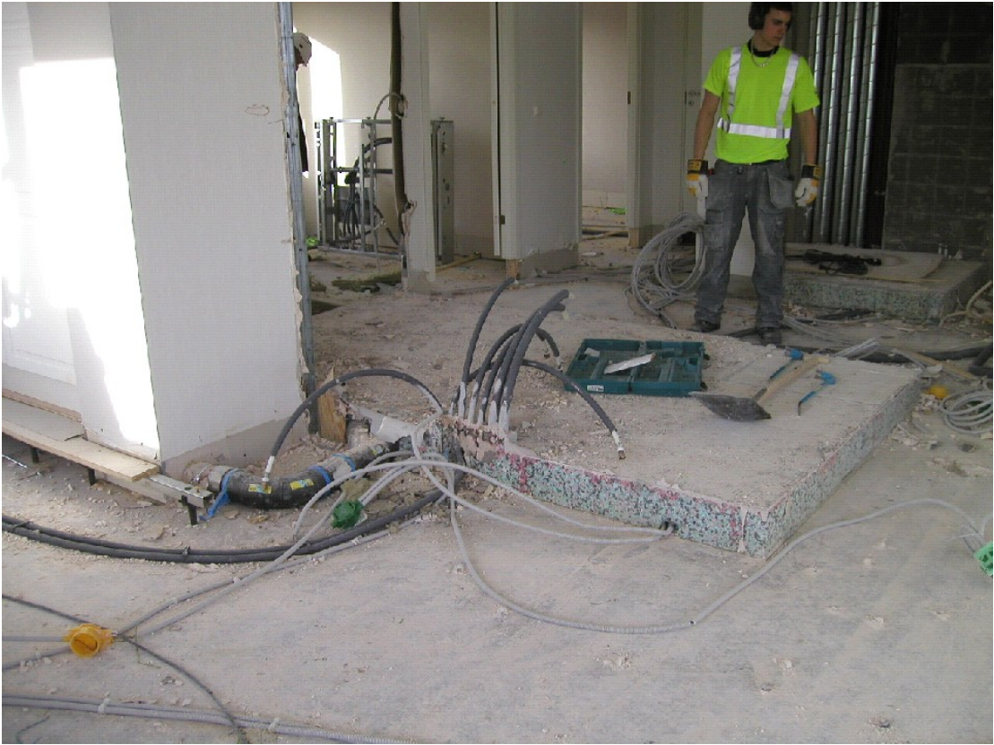
The similar view during stripping out of internal floors and other fittings
