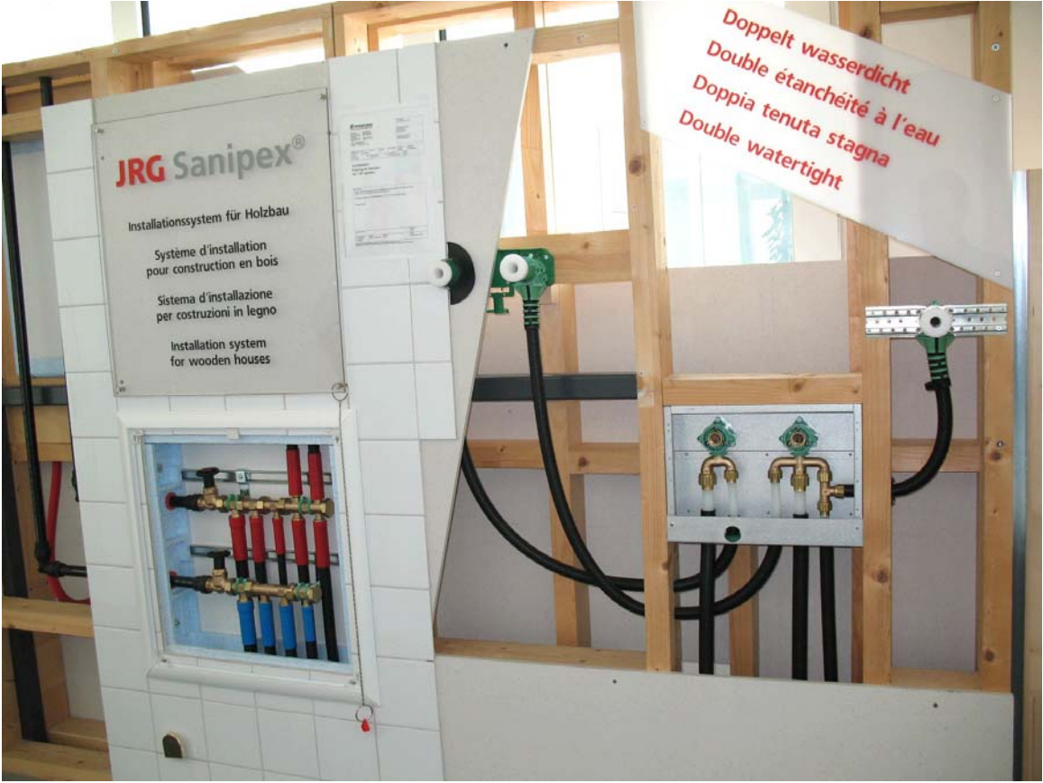
The principal lay out of an installation of a pipe in pipe system in a wooden frame house showing also a sample of the components needed.
