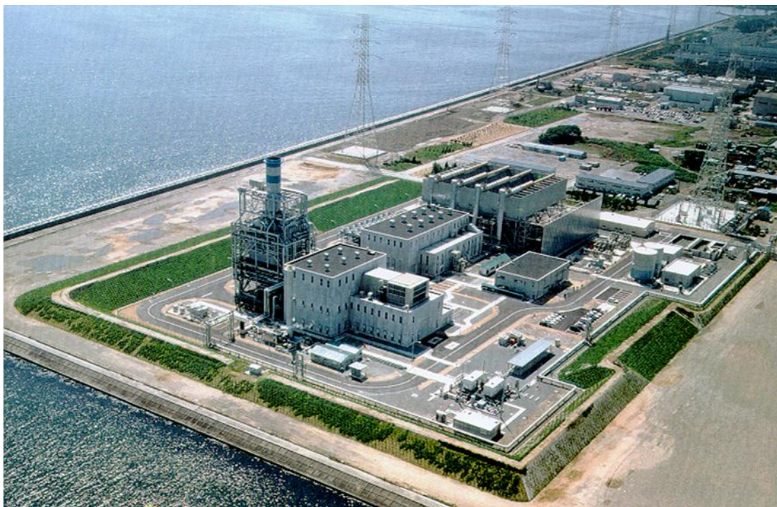
Figure 2. T-Point Validation Combined Cycle Power Plant.
