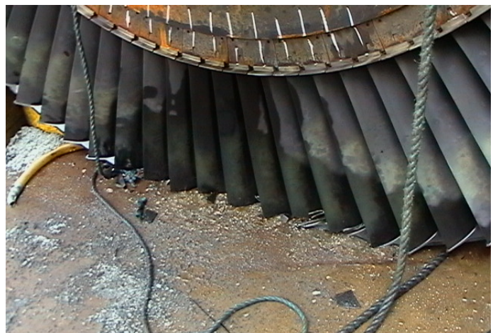
Turbine end hitting the ground
