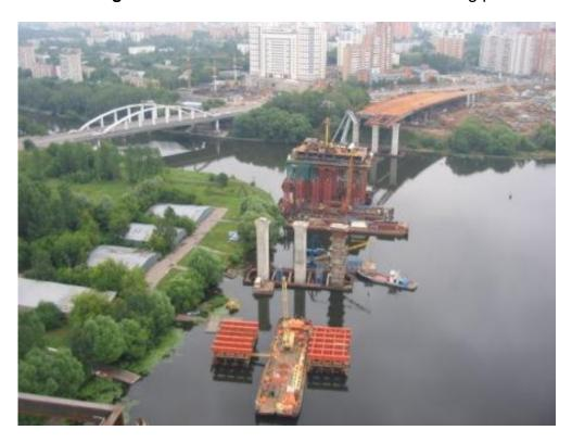
The arch pylon structure was assembled by the semi-cantilever method. As soon as the pylon is built and the superstructure is launched, the cable system consisting of 72 ropes to hold the superstructure to the pylon was installed.
