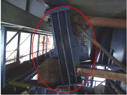
The main cause of the accident is excessive friction while moving the superstructure over the rolling facility in the course of launching, the friction having grown owing to pollution of the rolling ways with abrasive materials used while cleaning the superstructure and the pylon steel surfaces. And this was due to the personnel's negligence in removing the cleaning waste material from the rolling tracks. Besides the BO4 right temporary support also other temporary supports suffered damage.
