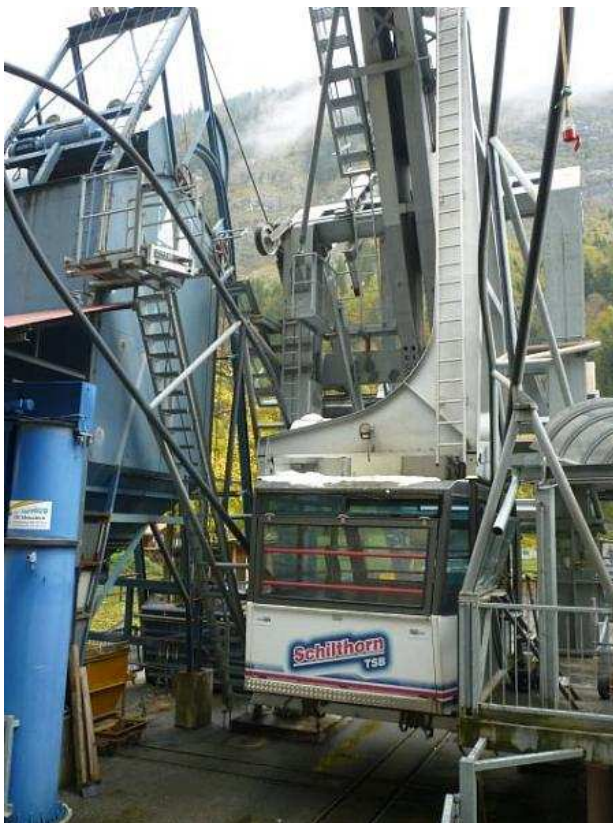
Valley station of Schilthorn cableway
