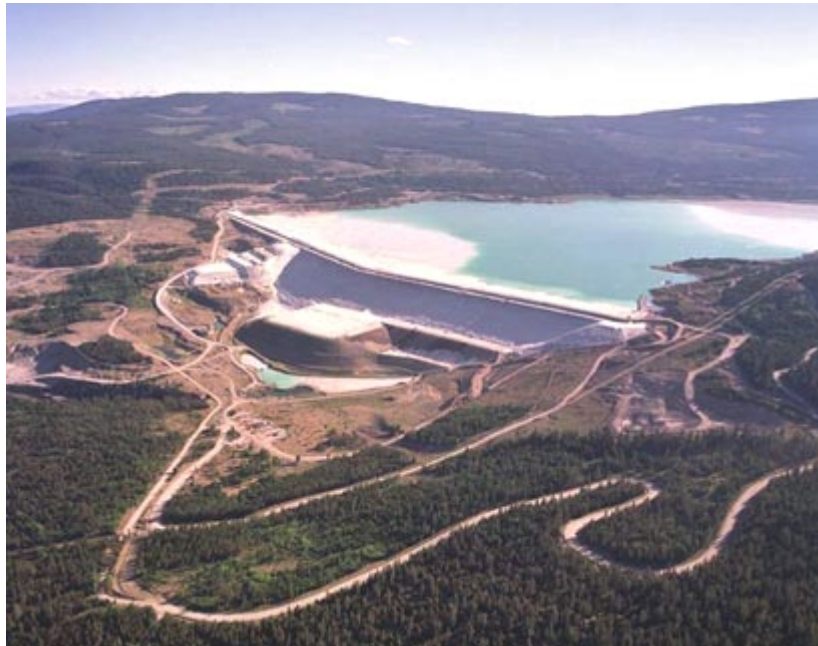
Cross valley tailings impoundment at Highland Valley Copper, BC, Canada (Courtesy TeckCominco)
