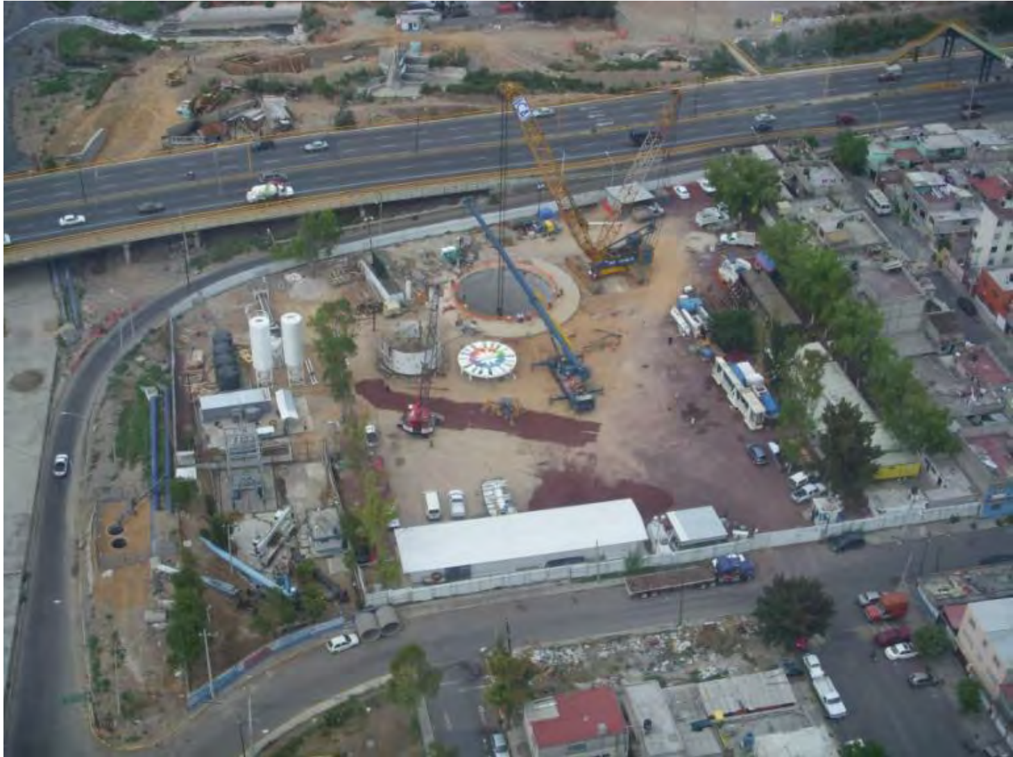
SHAFT 10. EMISOR ORIENTE TUNNEL. 2006
