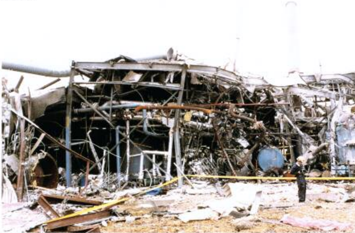
Part of the factory most severely damaged by the explosion
