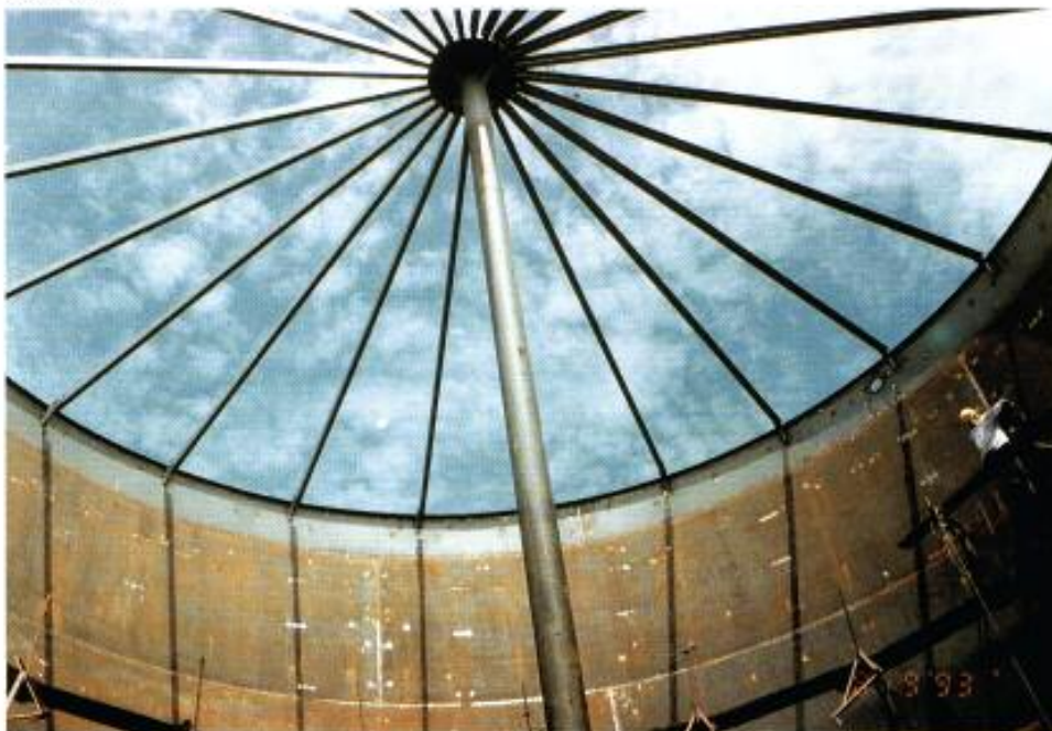
Tanks with an arrangement of roof beams between the upper rim and centre post were unaffected.
