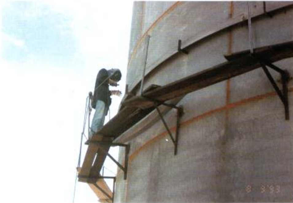
Fixing of wind girder along the fourth ring tank shell
