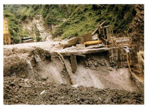
Slide No. 202 CPE and tunnel liner plates washed into the river-bed
