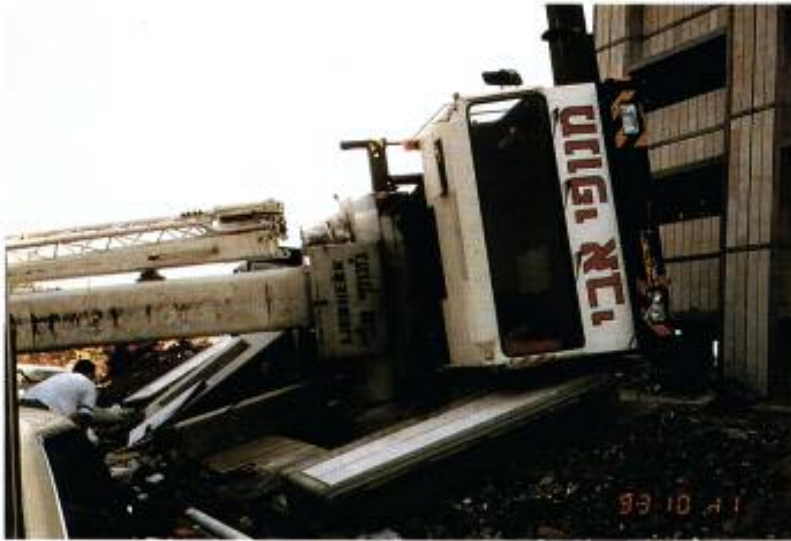
Clearly visible weak wooden planks on soft ground
