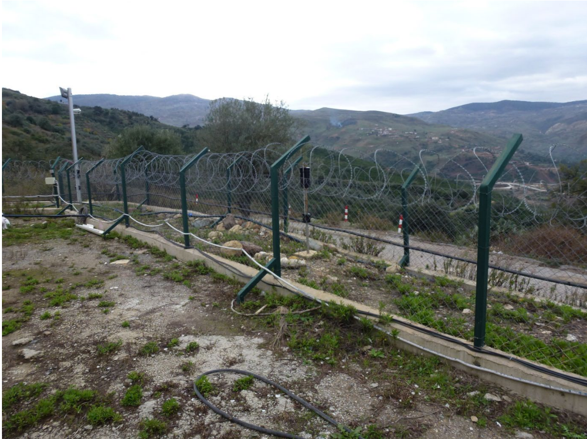
Site camp perimeter double fence with cameras and movement sensors
