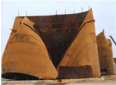
Fig. 14: Tank farm after windstorm [© MR]
