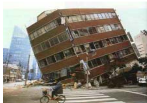
Fig. 30: Damage by Kobe-Earthquake 1995 [UNESCO.org]
