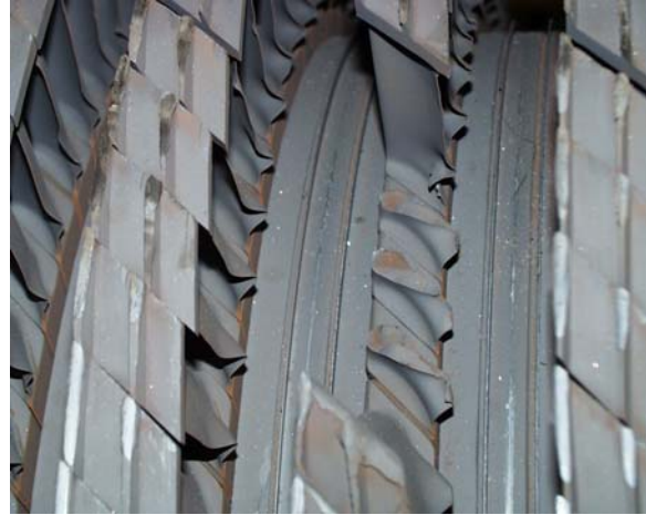
Water Induction Rub Compounded by Attempts to Turn Thermally Locked Rotor
