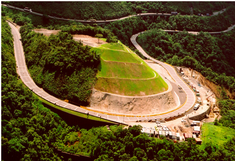
Photo No. 4: View of Via Anchieta Highway after repair completion
