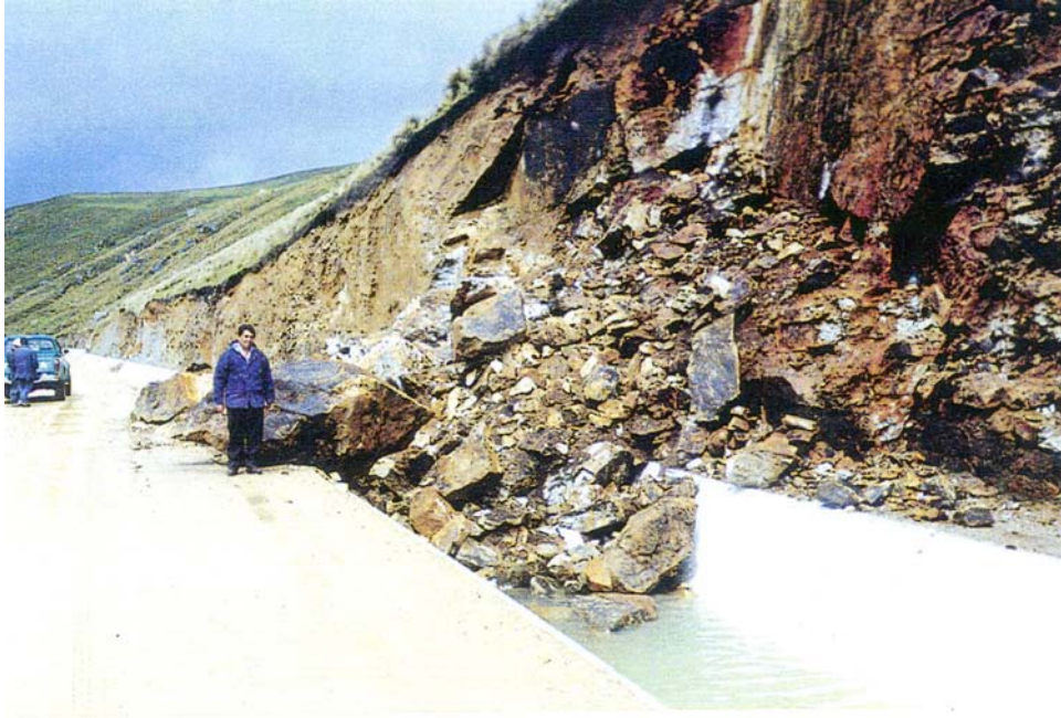
Photo No. 2: Debris deposited on works, after loss
