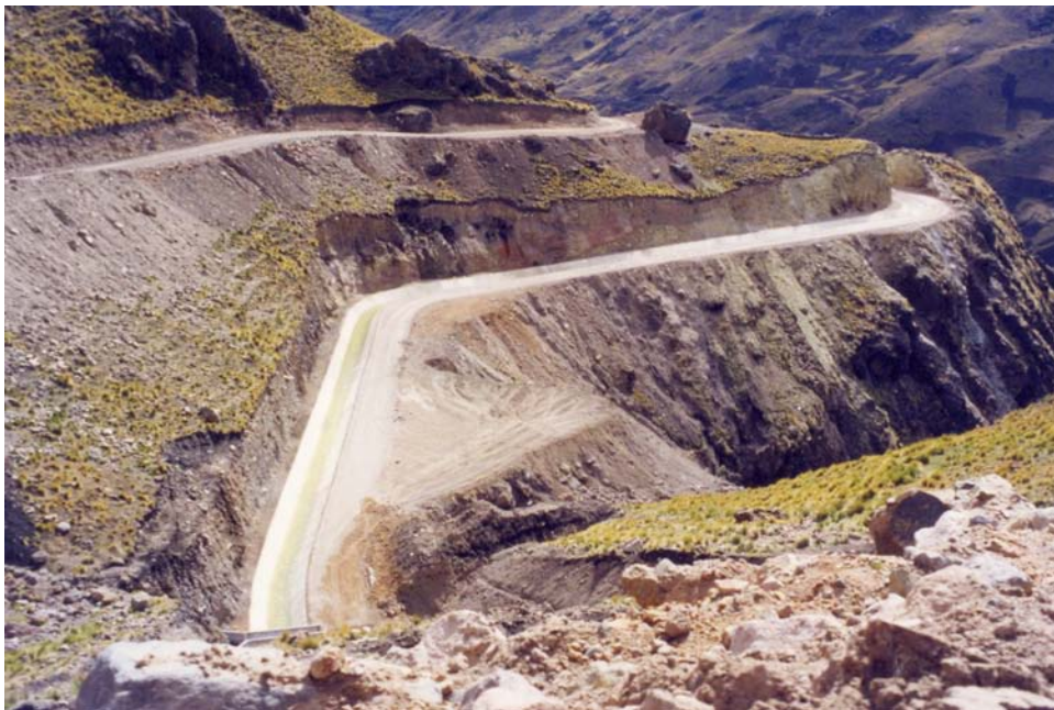
Photo No.1: Road and canal construction prior to loss
