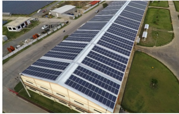
No air gap (not acceptable)
