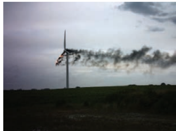
Fig. 1: Fire after lightning struck a 2 MW wind turbine in 2004 ( Image source: HDI/Gerling )
