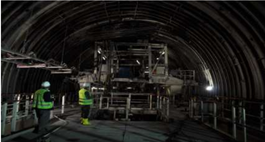
Fig. 2: Continuous application of stiff support as to enable excavation with the TBM
