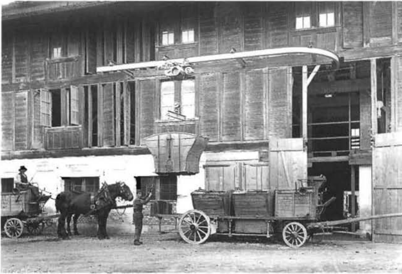
Domestic refuse collection carts using transportable containers. Zurich's municipal cleansing department used these carts in the period 1910–1930.
