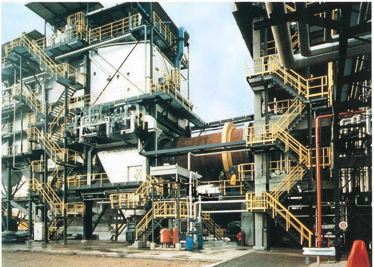
Rotary kiln in an incineration plant for hazardous waste
