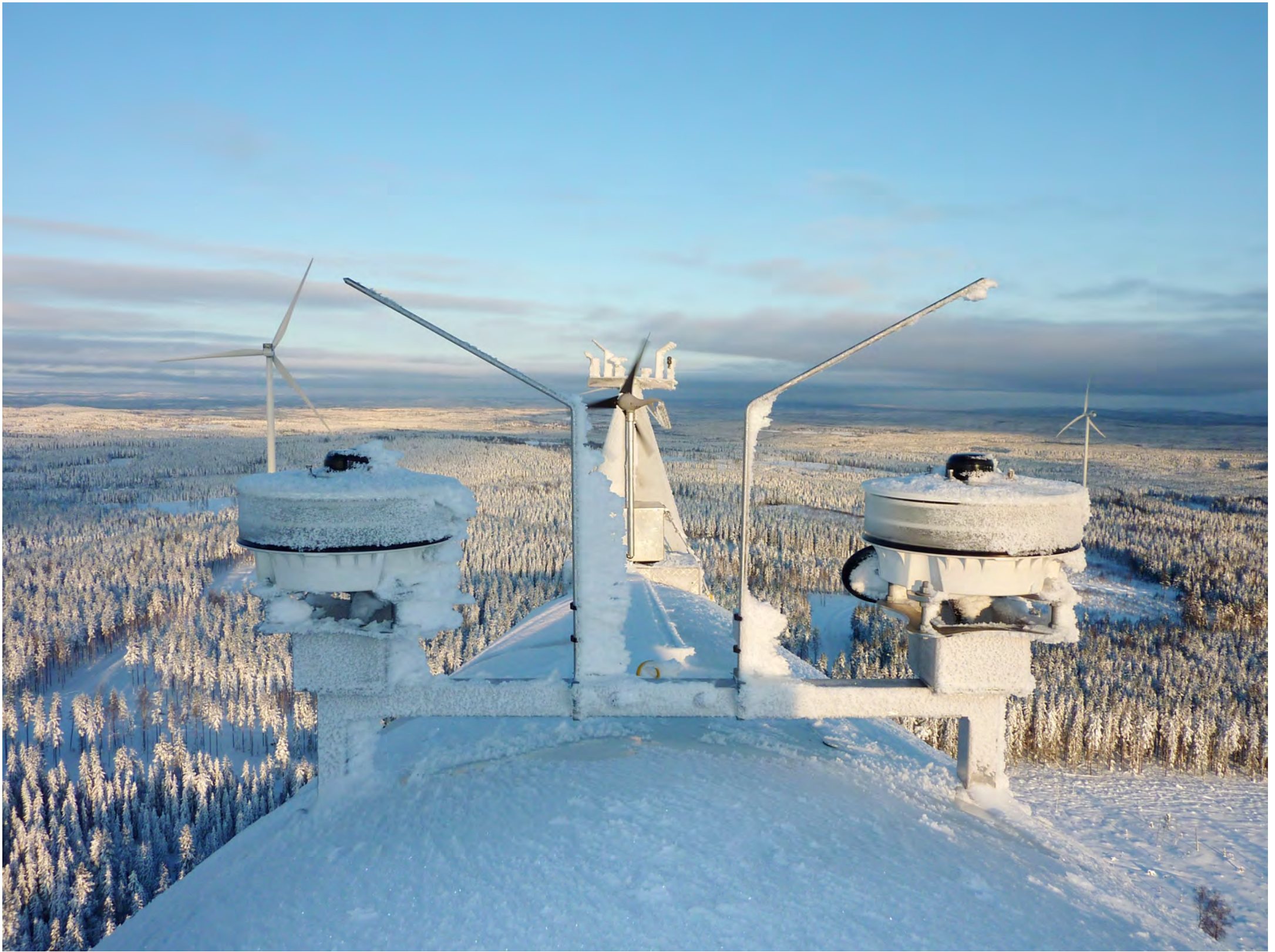
Measuring device on a wind turbine of a wind farm in Sweden seen at -20 C (Gernot Löschenkohl, Munich Re)
