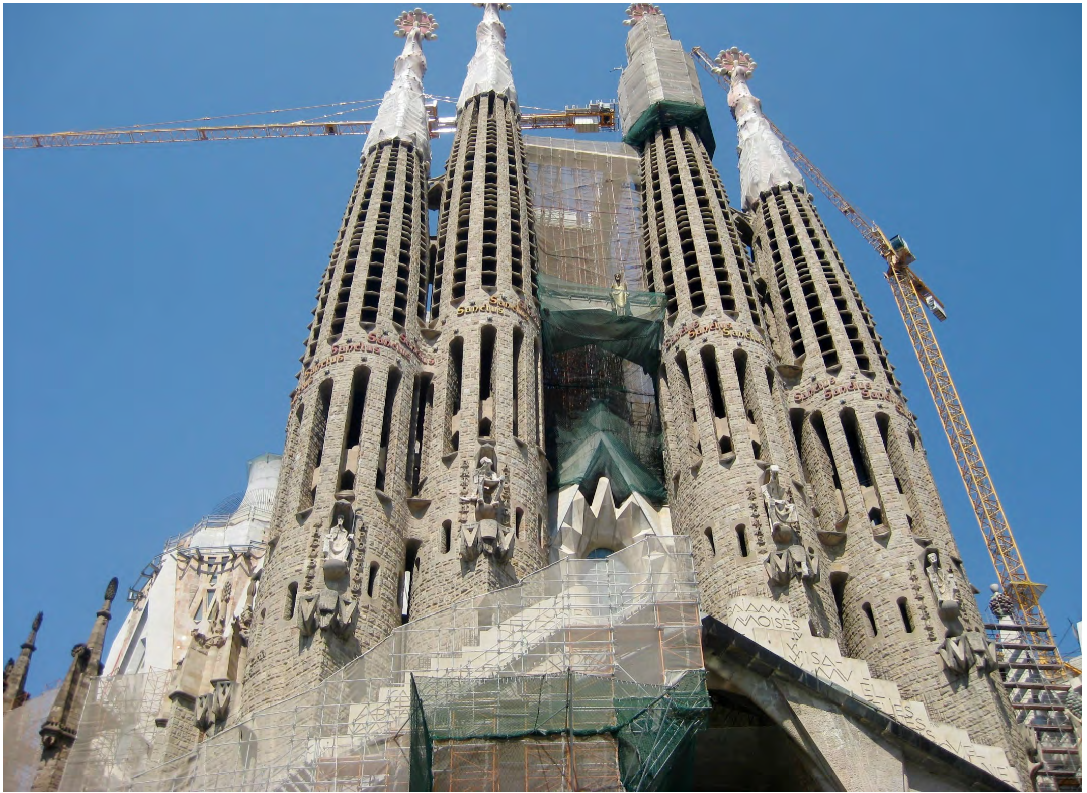
On-going construction of the Basilika Sagrada Familia – Barcelona (Christoph Hoch, MRe)
