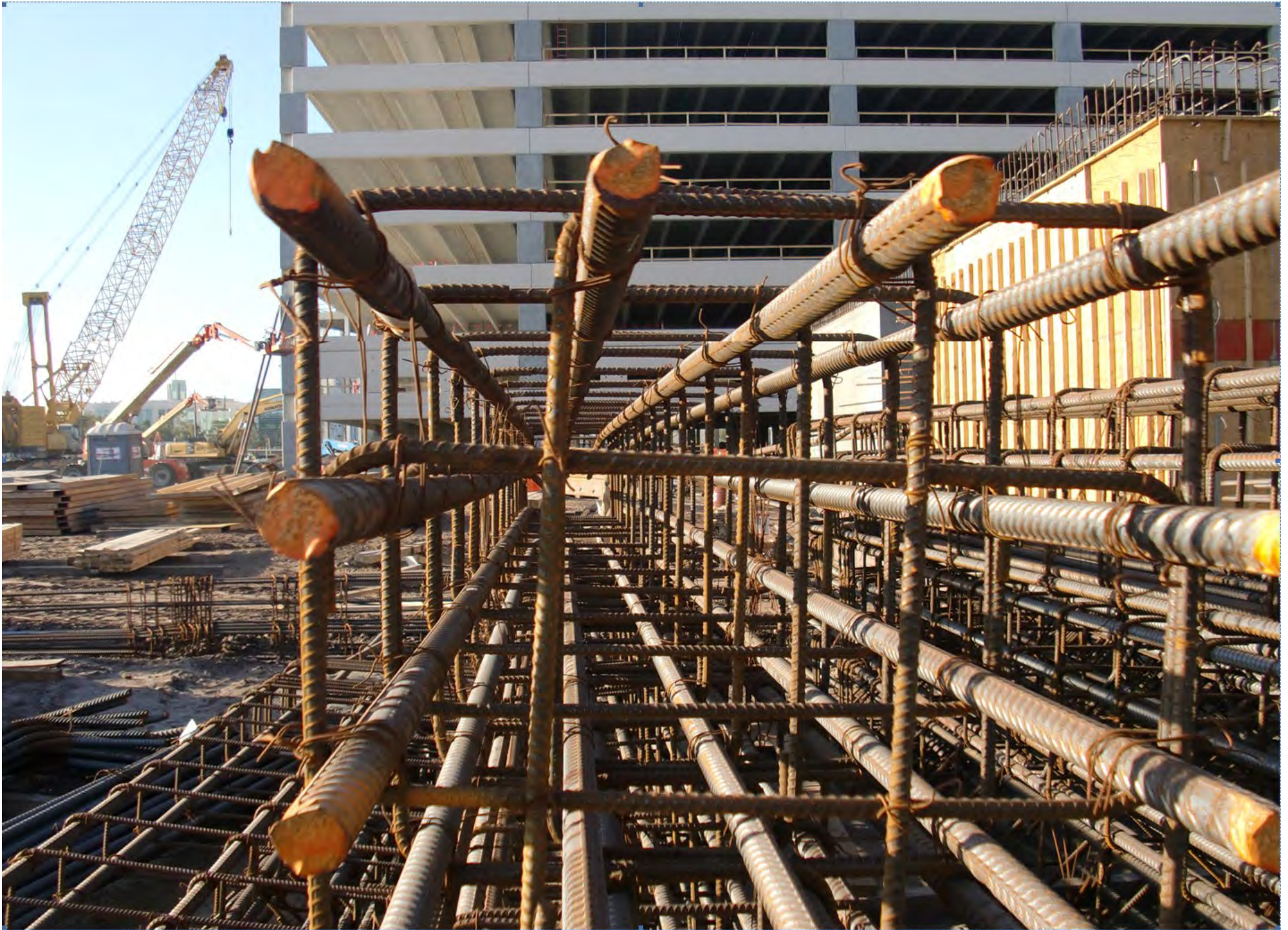
Construction of Orlando Hospital, USA (Gero Stenzel, Partner Re)
