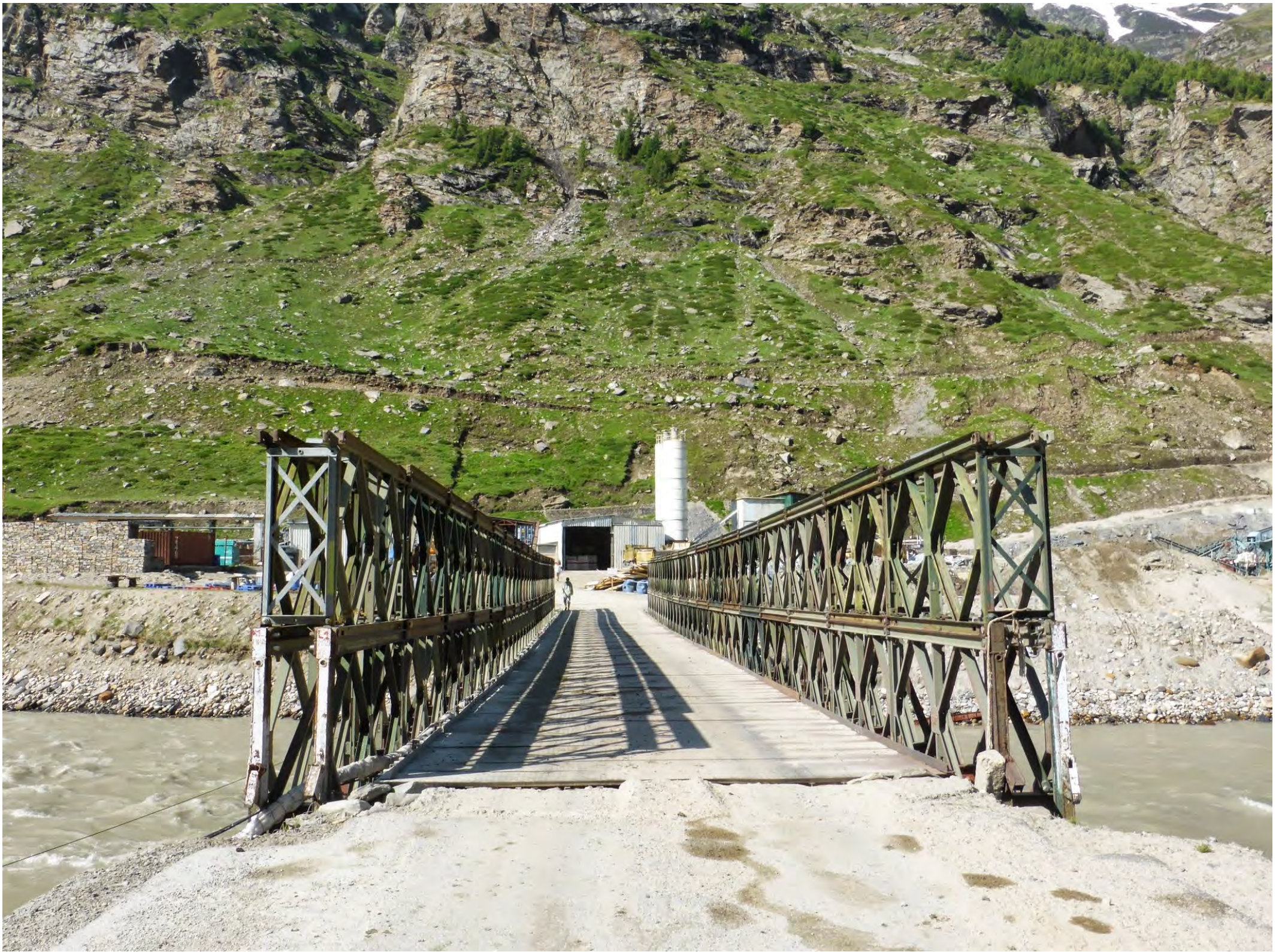
Steel bridge in India (Frank Ruopp, Munich Re)
