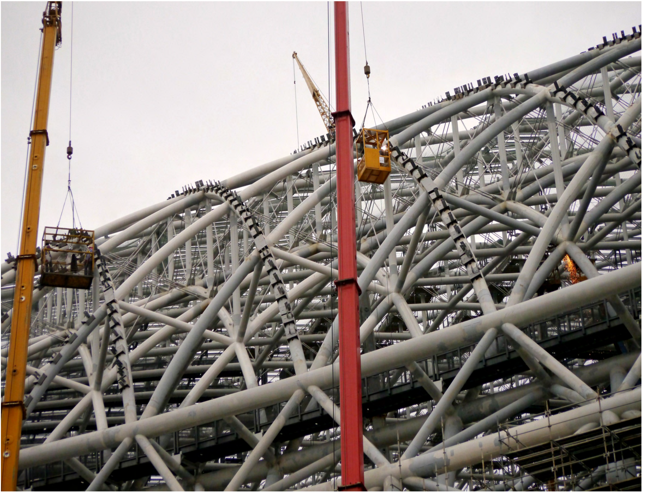
Taipeh New Area Construction - by Simon Chen, Engineering Insurance Association
