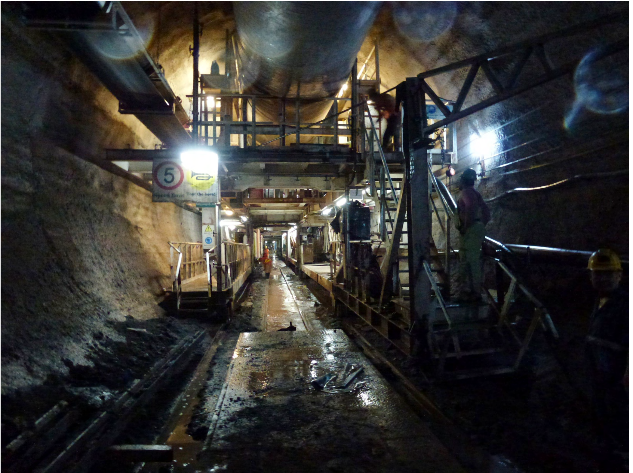
Tunnel boring machine – by Richard Radevsky, Charles Taylor Adjusters
