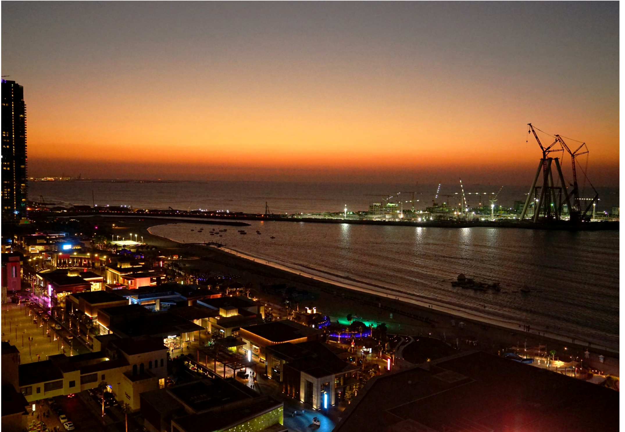
Construction of a giant wheel in Dubai - 2016 – Andy Hottinger, Axis Re
