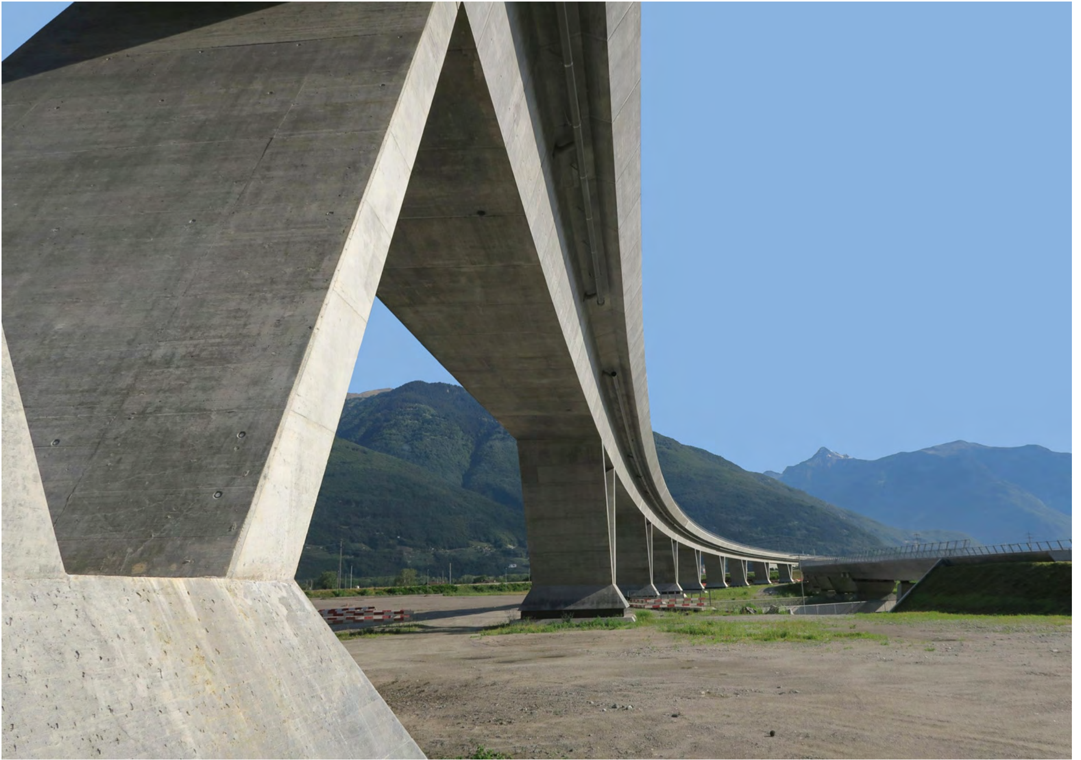
Access bridge at Ceneri Tunnel (1) – 2016 – Gero Stenzel, Partner Re
