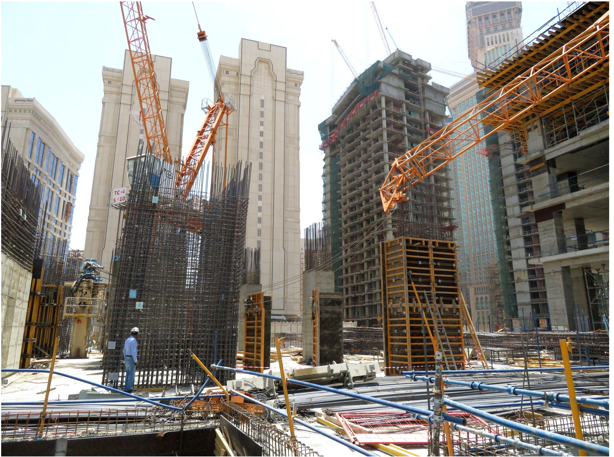
Construction Works in Mecca – 2016 – Mamoon Alyah, CEERISK Consulting
