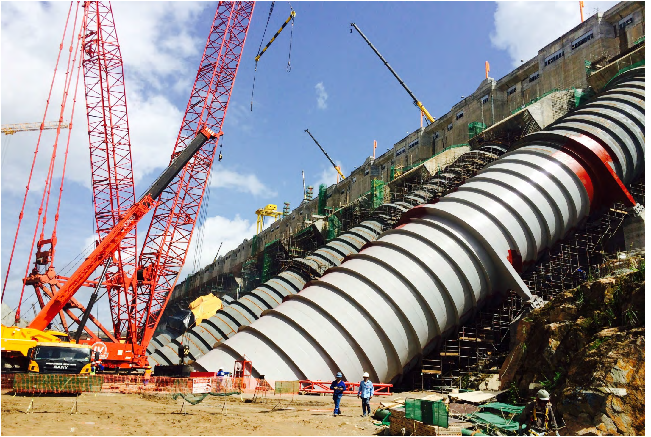
HPP Belo Monte – Penstock View - by Lucas Lopes Princeton New Jersey, USA (2017)
