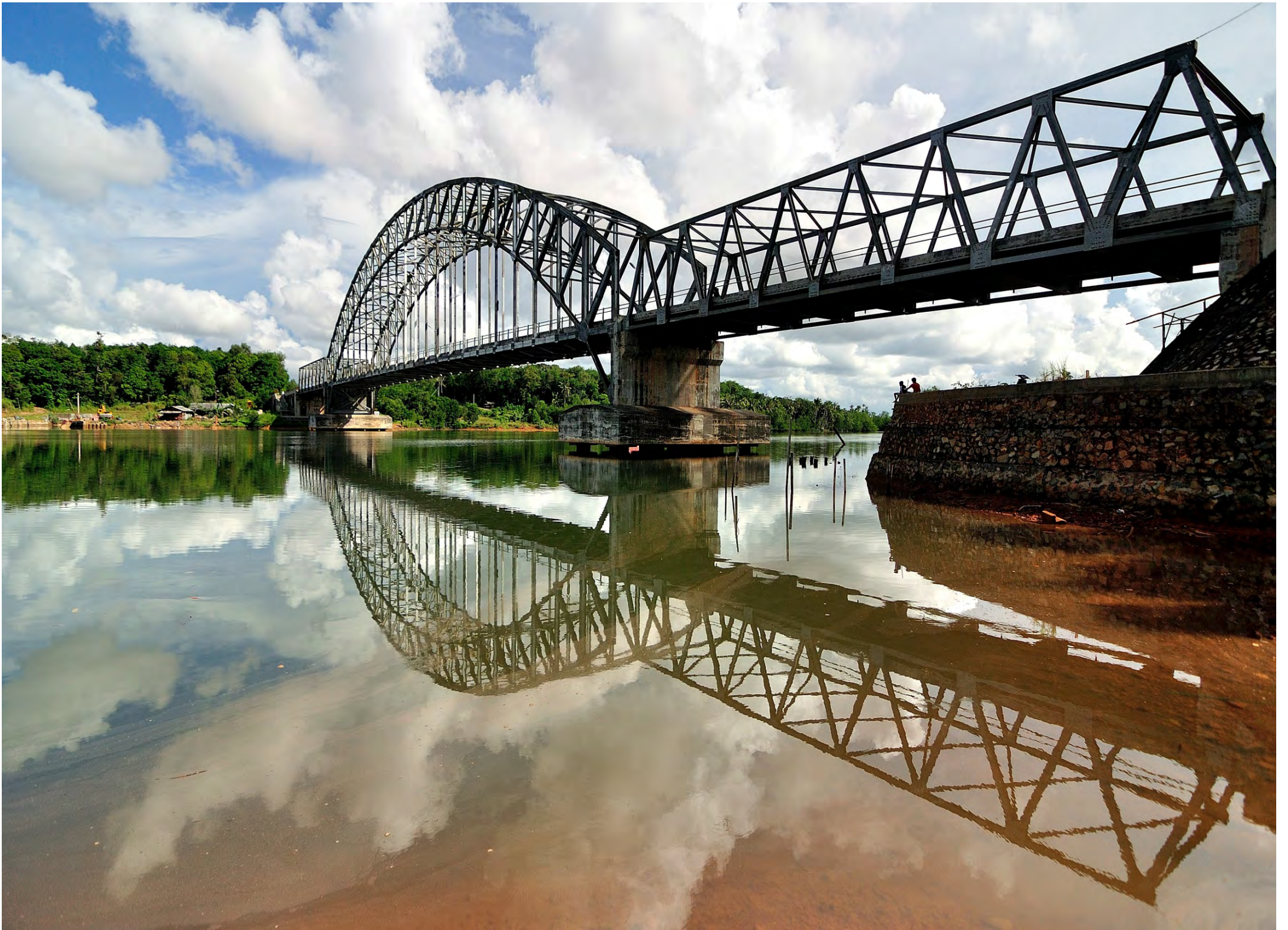
Railway bridge - by Deddy Hendrawan - Arizona USA (2017)
