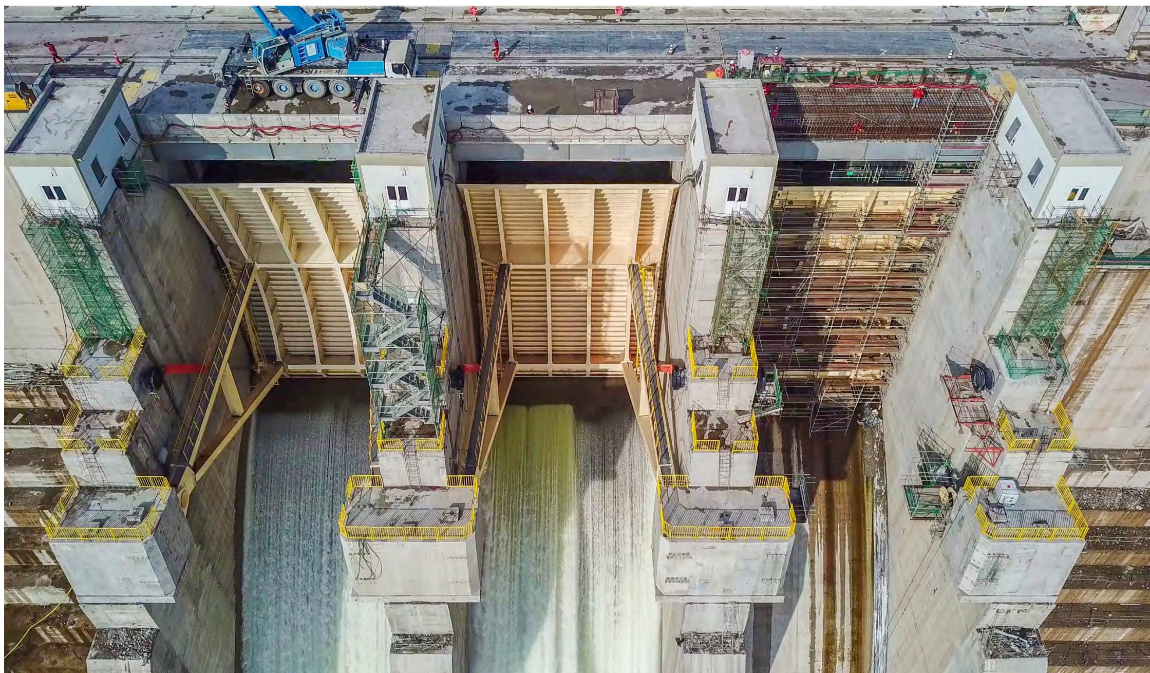
Hydro Power Plant Lauca – by Antonio R Peynau, Odebrecht (2018)
