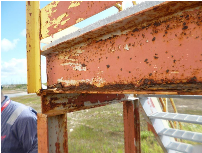
Corrosion visible and damaged coatings.
