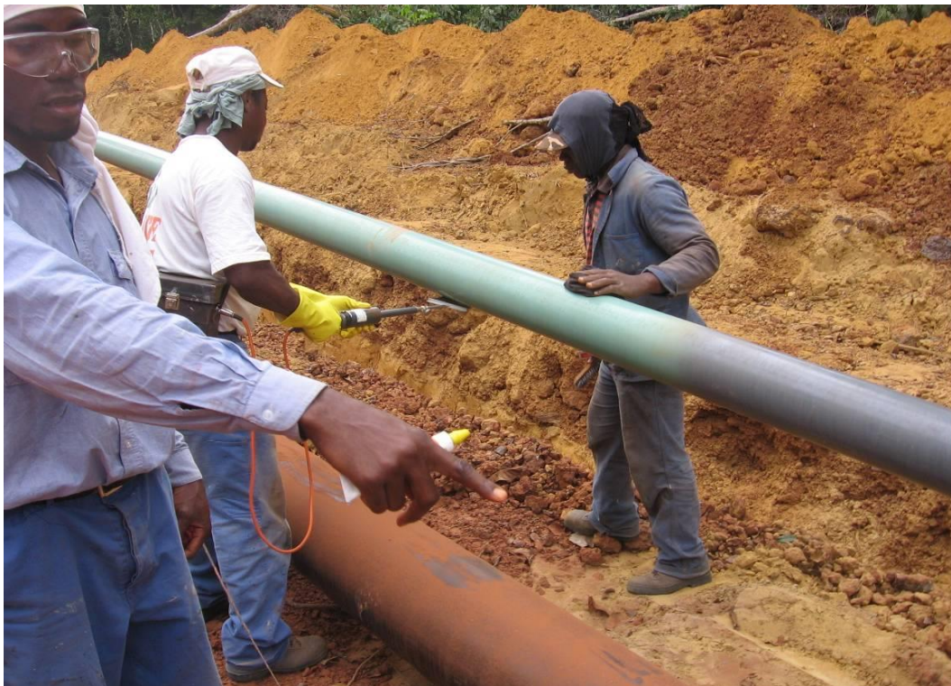
Checking coating integrity using a spark test on site.
