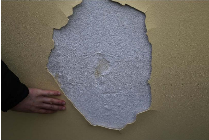
Picture 4: Detaching of paint and mushy render layer below
