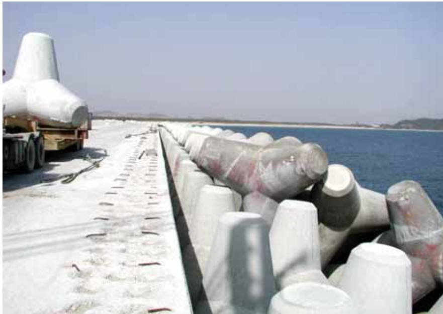
Tetrapods in front of a quay wall
