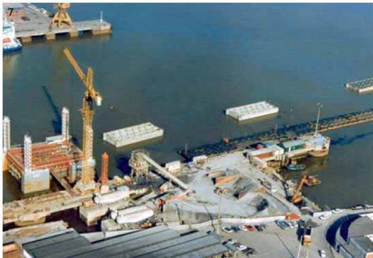
Floating caisson fabrication Illustrations MR
