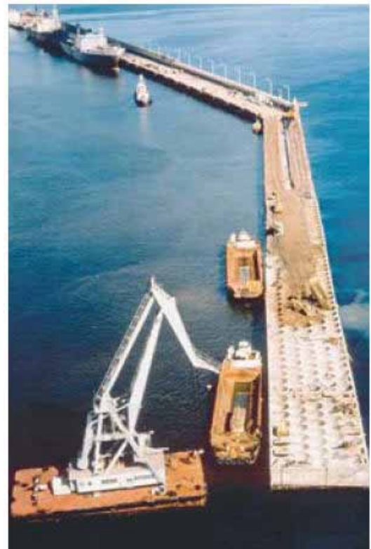
Placement of caissons
