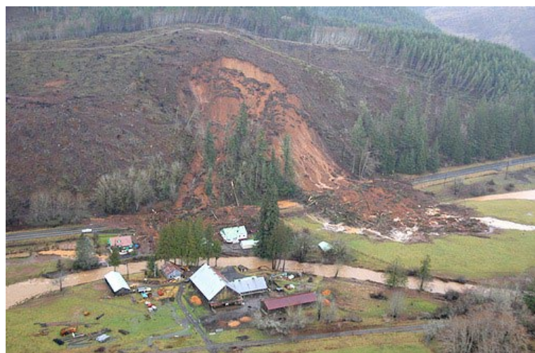
Mudslide due to heavy rainfall
