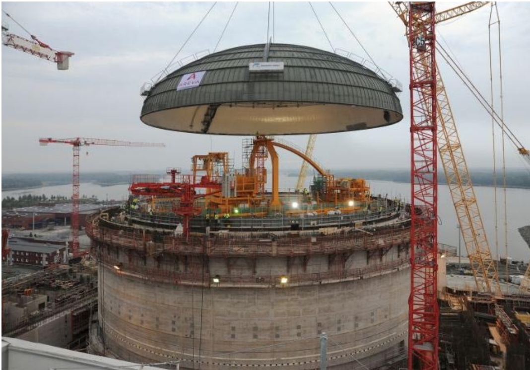
Critical construction operation: Lifting of large diameter dome onto reactor containment
