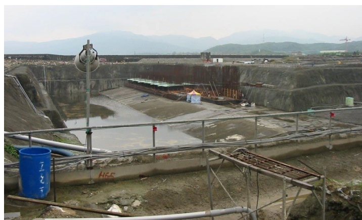
Construction of Cooling Water Pump Basin, slightly flooded
