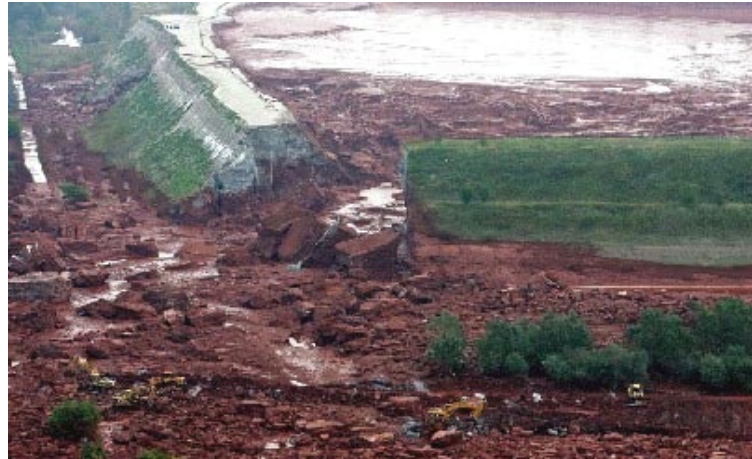
Failure of protection dam
