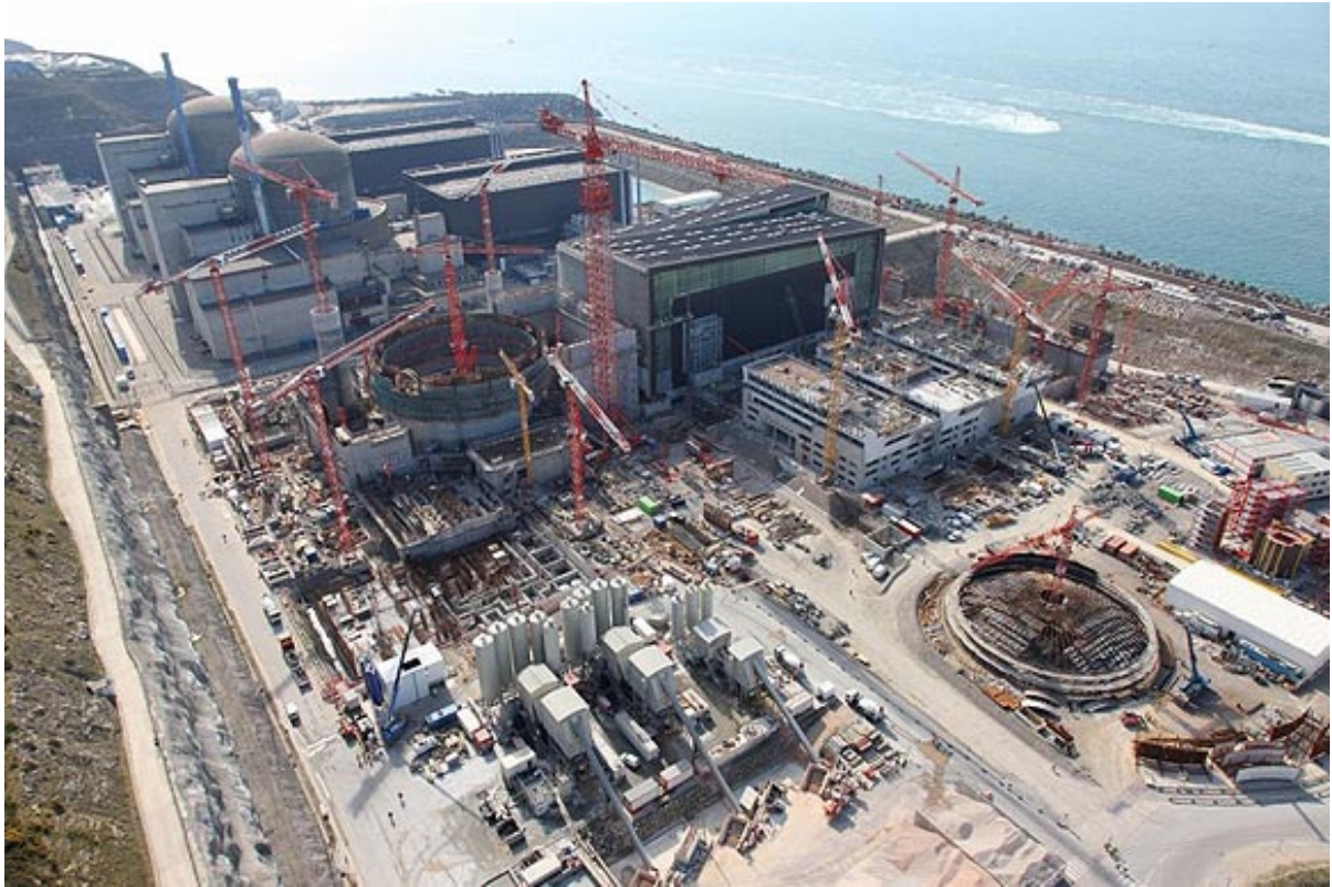
Flamanville EPR Construction site (source: Atominfomedia July 2011)
