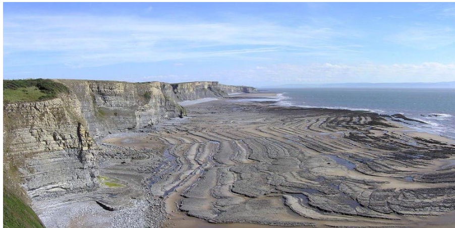
Soil erosion due the wind and wave action
