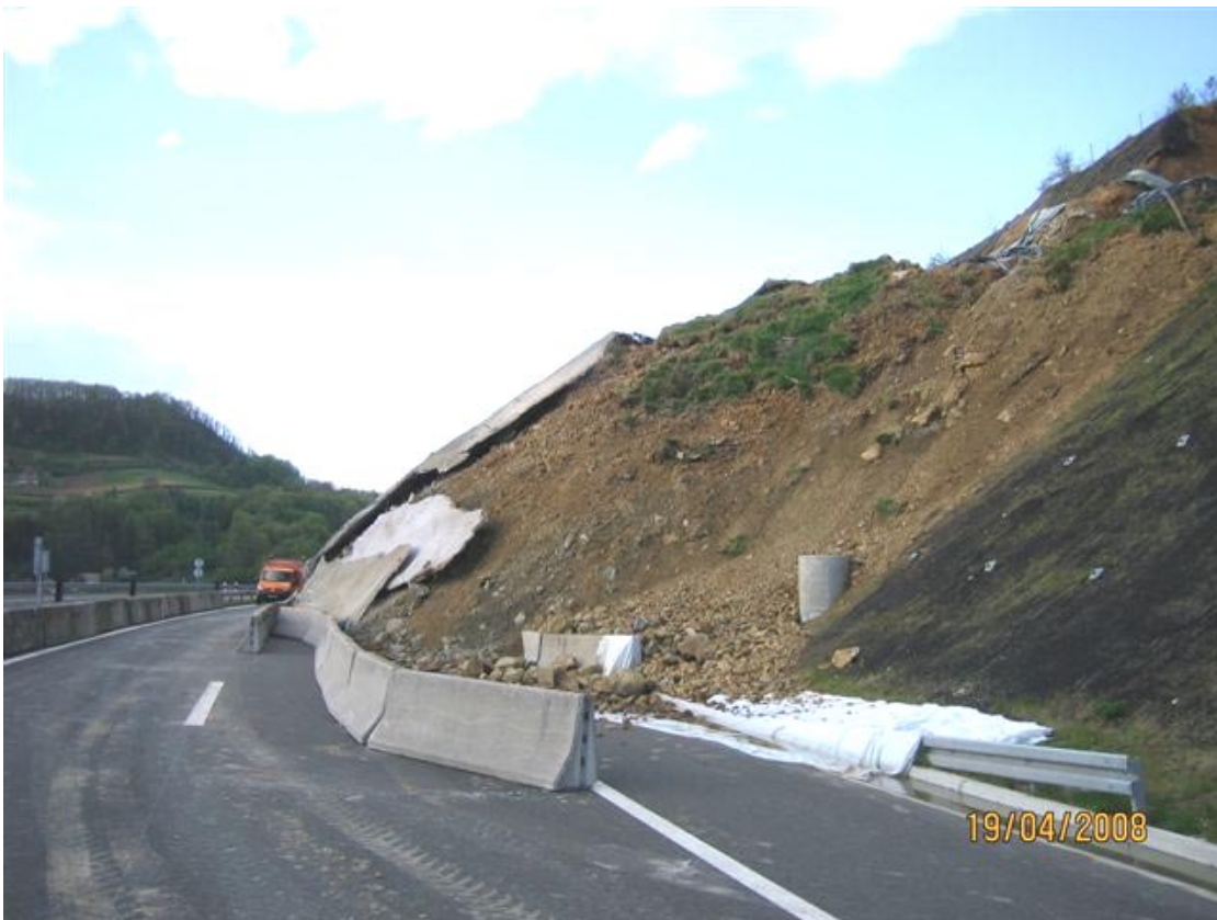
Situation shortly after the landslide occurred
