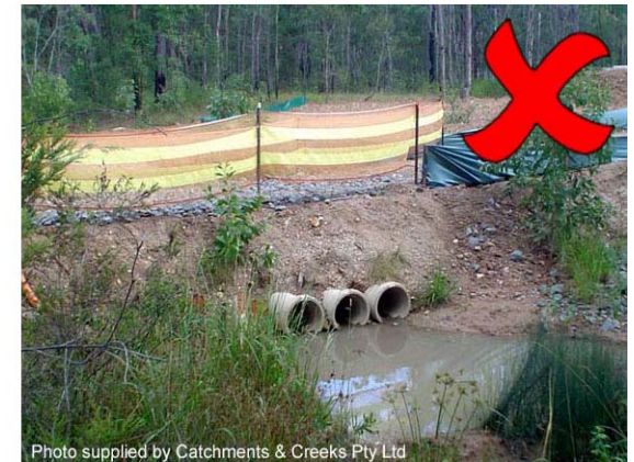
Photo supplied by Catchments & Creeks Pty Ltd
