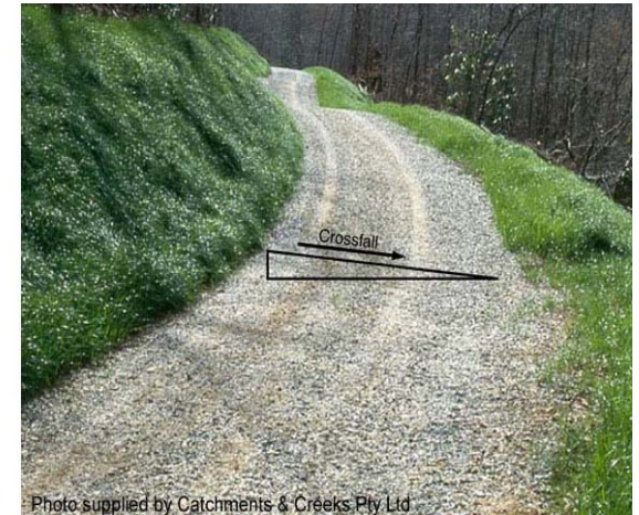
Photo supplied by Catchments & Creeks Pty Ltd
