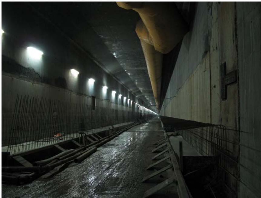
View inside the immersed tunnel
