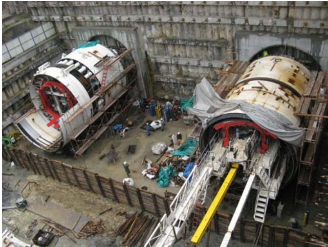
Refurbishing works for TBMs at Yenikapi Station
