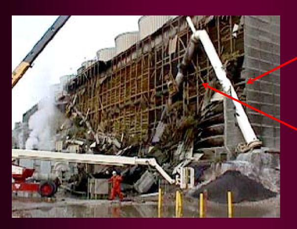
Riser which was possibly pulled by the collapsing Distributor
