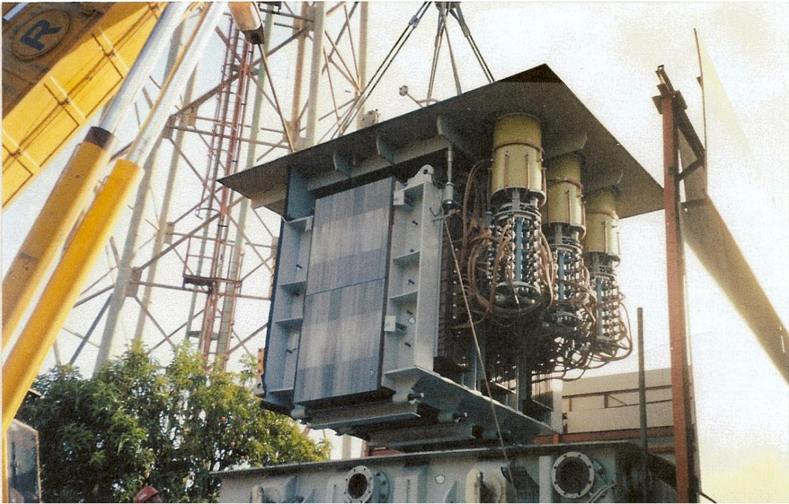
Picture 1 shows the disassembling activities
